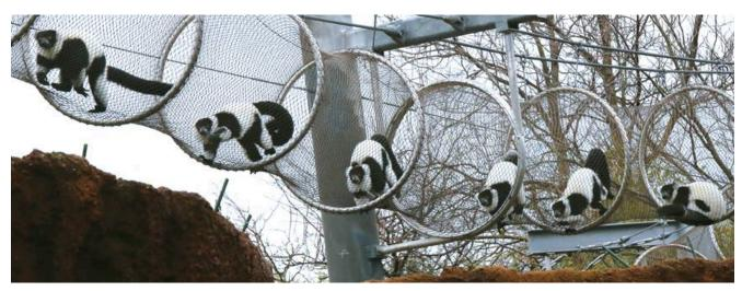
The structure of the stainless steel cable wire mesh net is a grid structure. If the size of the monkey is relatively large, a large mesh can be selected, and the wire rope is relatively thin. It is conceivable that the perspective of the fence is very good.
